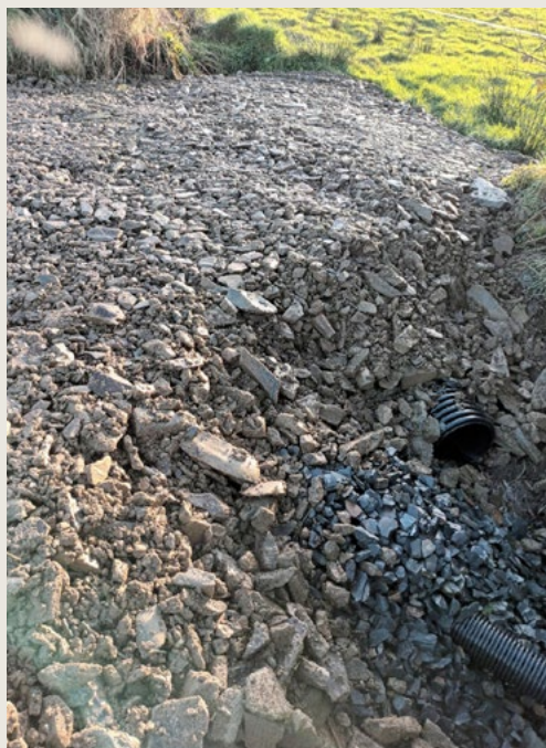
Pictured left: A Sustainable Crossing Point reducing sedimentation in a farm drain.
