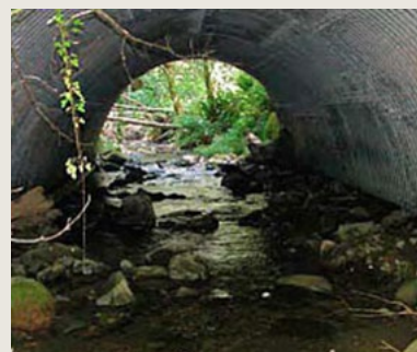
Pictured left: A Sustainable Crossing Point reducing sedimentation in a farm drain.
